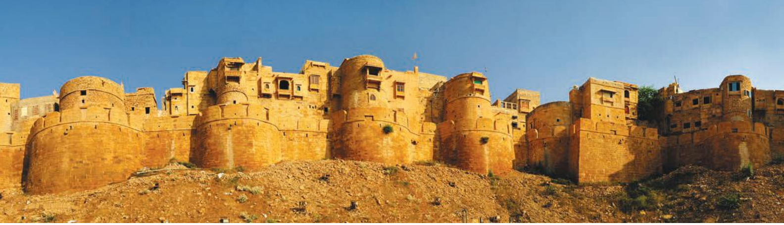
Fig. 1.18. Jaisalmer fort, Rajasthan. A mud structure built in the 12 th century and refurbished later using sandstone.
