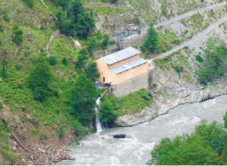
Fig. 1.2. A microhydel plant in Himachal Pradesh—the power of flowing water converted into electricity
