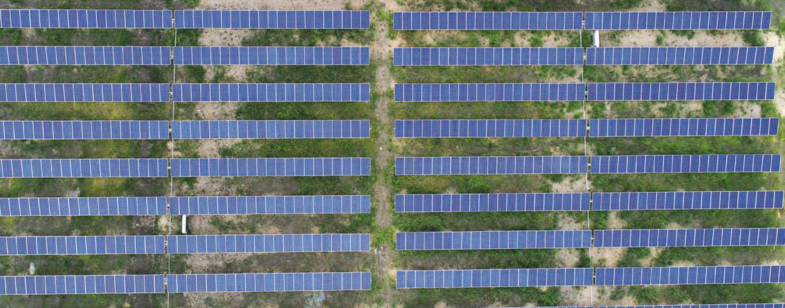
Fig. 1.22. Solar farm near Raichur, Karnataka
