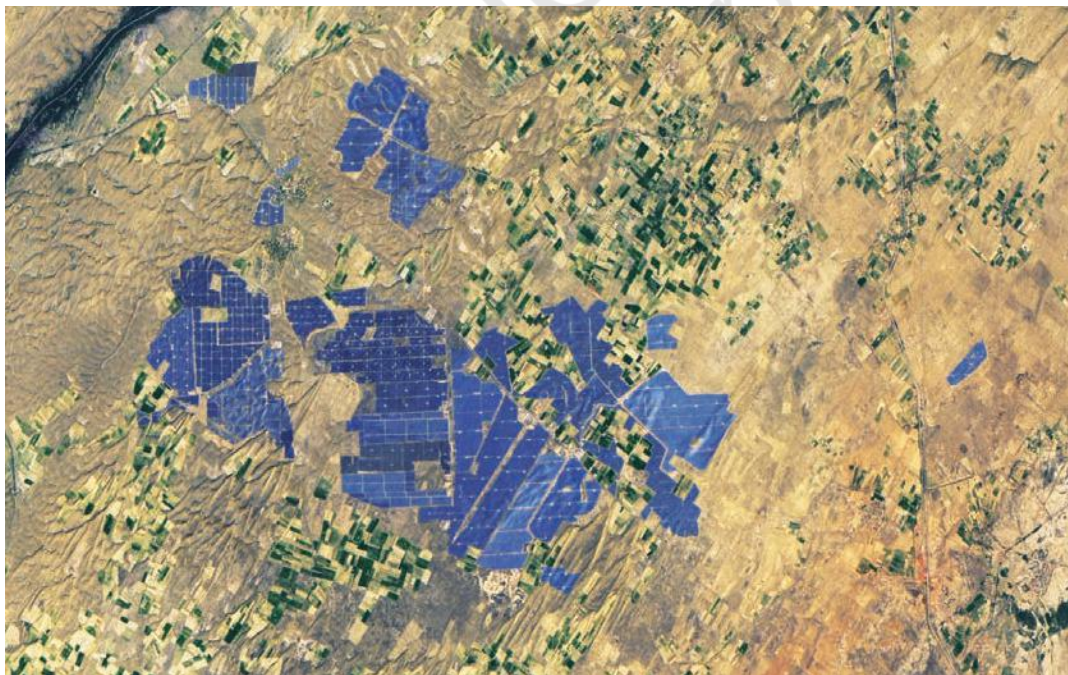
Fig. 1.21. Satellite image of one of the largest solar parks in the world located in Rajasthan. It can generate enough electricity to power about 15% of the current needs of Rajasthan.
