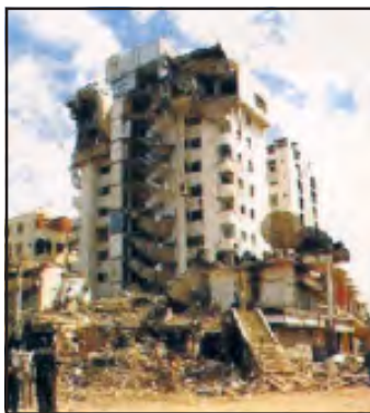
Fig. 3.3a: Destruction caused by an Earthquake in Gujarat
