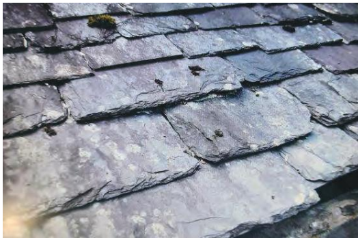
Fig. 11.6: Rocks used for roofing
