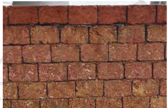
Fig. 11.7: Laterite rocks used as bricks
