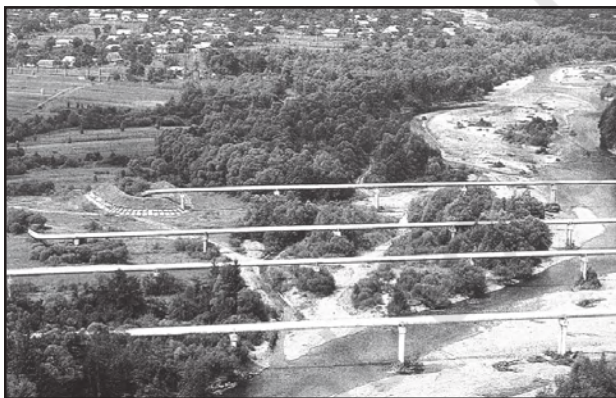
Fig. 7.17: Pipelines transporting natural gas in Ukraine
